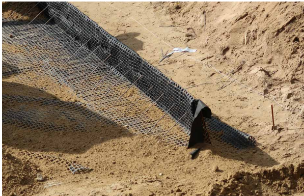
Geogrid reinforcement in a bridge construction.
