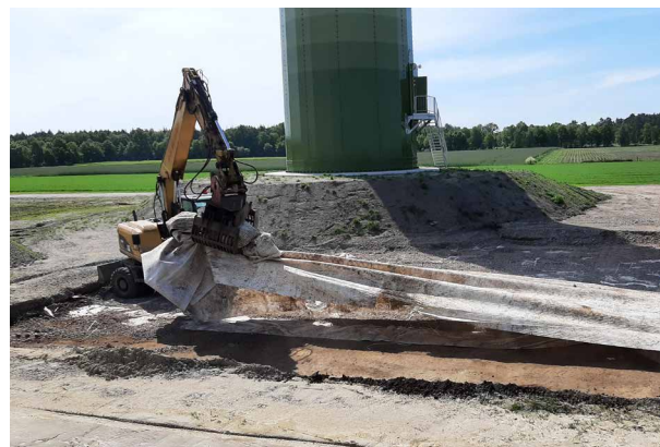
Deconstruction of a geosynthetic.
